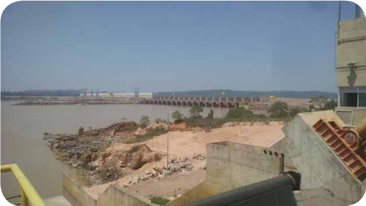
Figure 1: Jirau hydroelectric power plant is among the largest hydropower plants in the country
