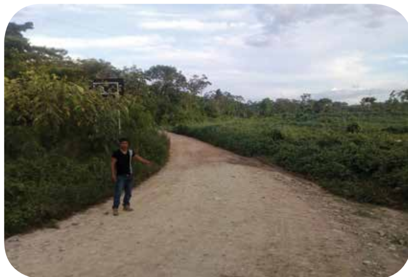
Photo 2. Road to be improved in the Prioritized Project
